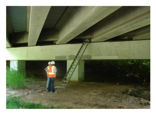
Figure 3.2.1: Girder access shown for Silver Comet Trail bridges, Structure ID 067-5186-0, in Cobb County
