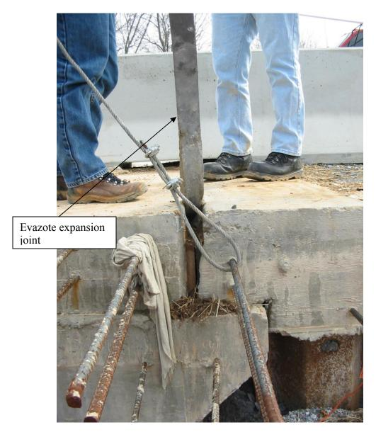
Figure 1.5.2: Evazote expansion joint during installation
